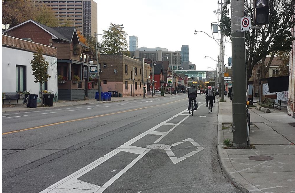
Permanent Buffered Bike Lane Markings
