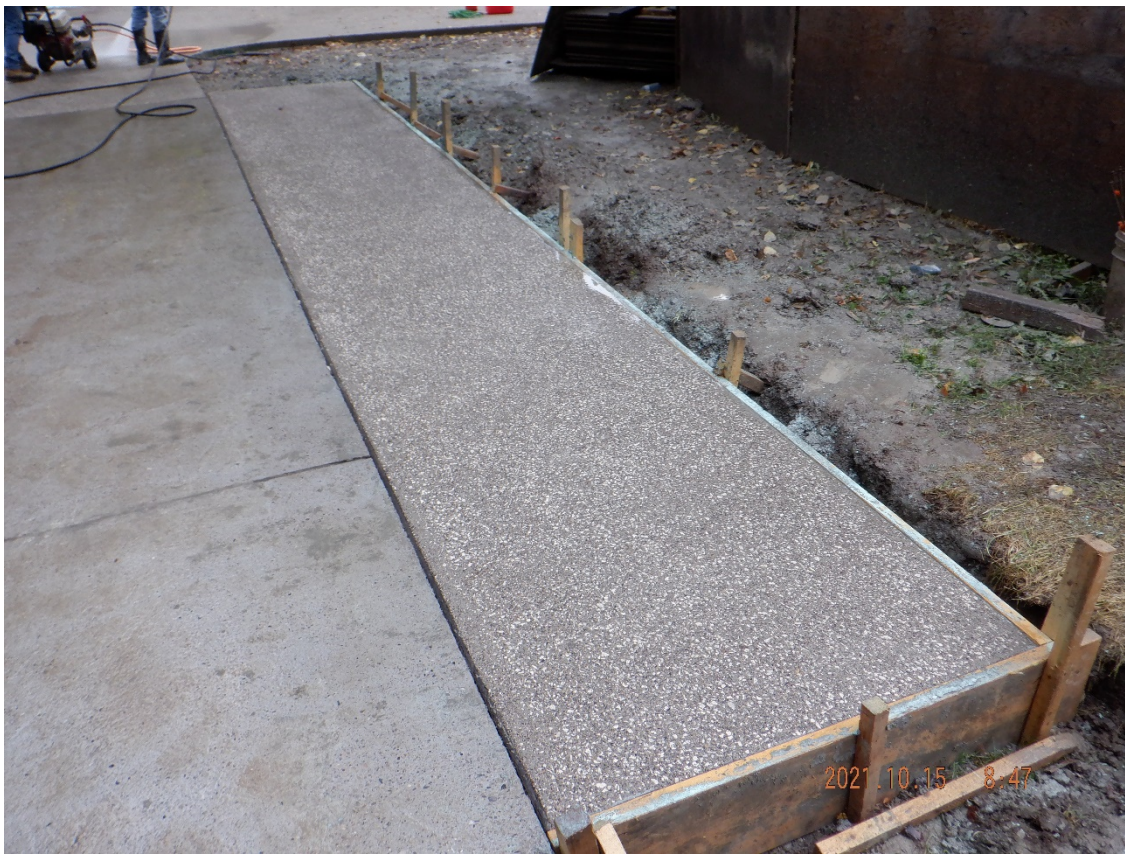
Concrete pad for the garbage enclosure near the Valve House in Little Park/Summerhill Entrance
