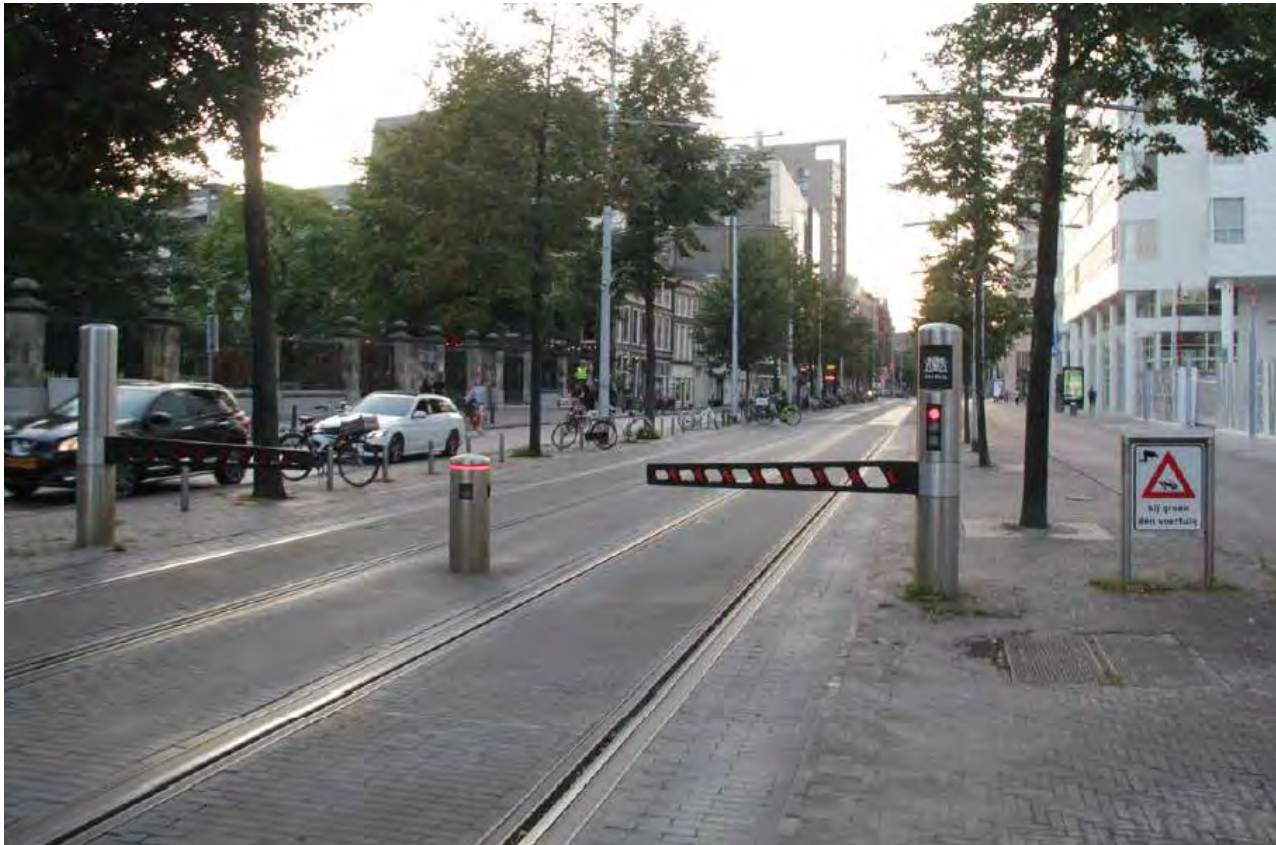
Example of automated gate, Den Haag, Netherlands
