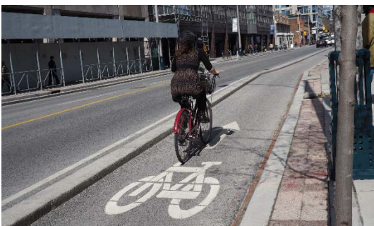
Example of physically separated (concrete curb) street-level bike lanes (cycle tracks) on Wellesley Street
