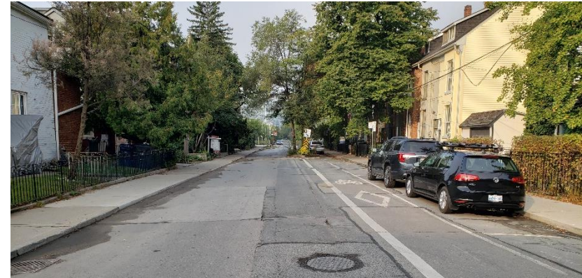
Wellington St at Tecumseth St – looking west
