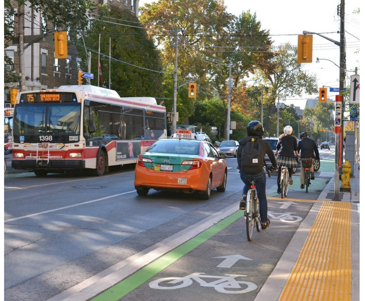
Integrated raised cycle track at a TTC bus stop on Sherbourne St
