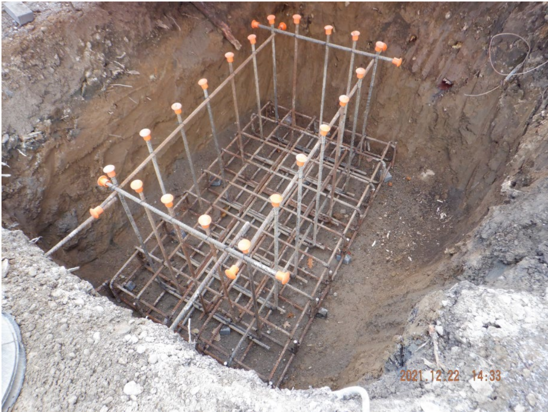
At Avoca entrance node: formwork and reinforcement for foundation of the Heritage Valve (public art)
