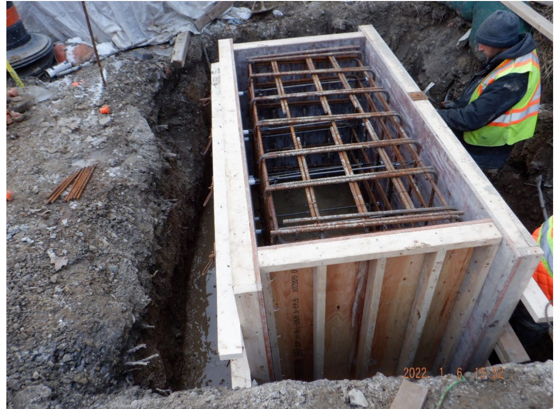
At Avoca entrance node: formwork and reinforcement for foundation of the Heritage Valve (public art)
