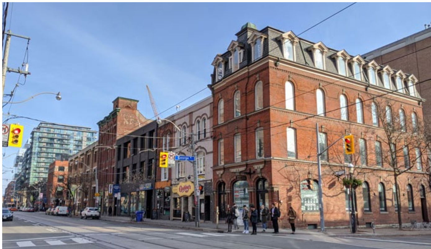
Figure 17: The streetwall along King Street East is a strong example of uniform setback and roof lines
