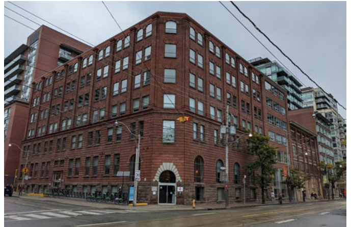
Figure 12: 204 King St. East, an example of Industrial Building Typology
