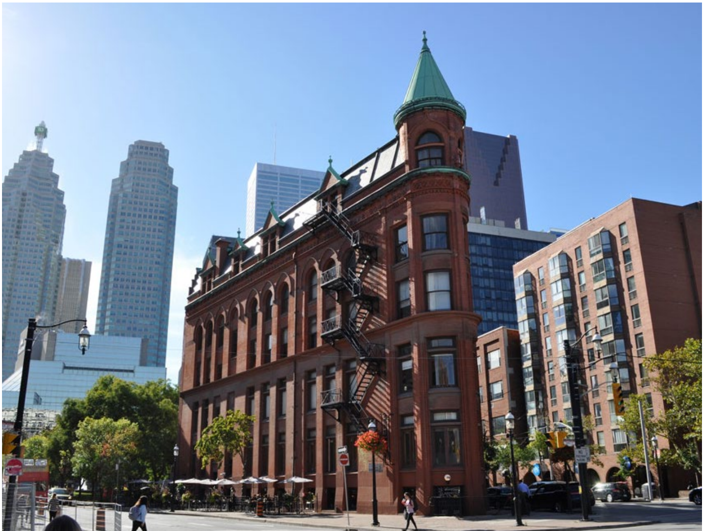
Figure 23: 49 Wellington St. East, the Flatiron Building
