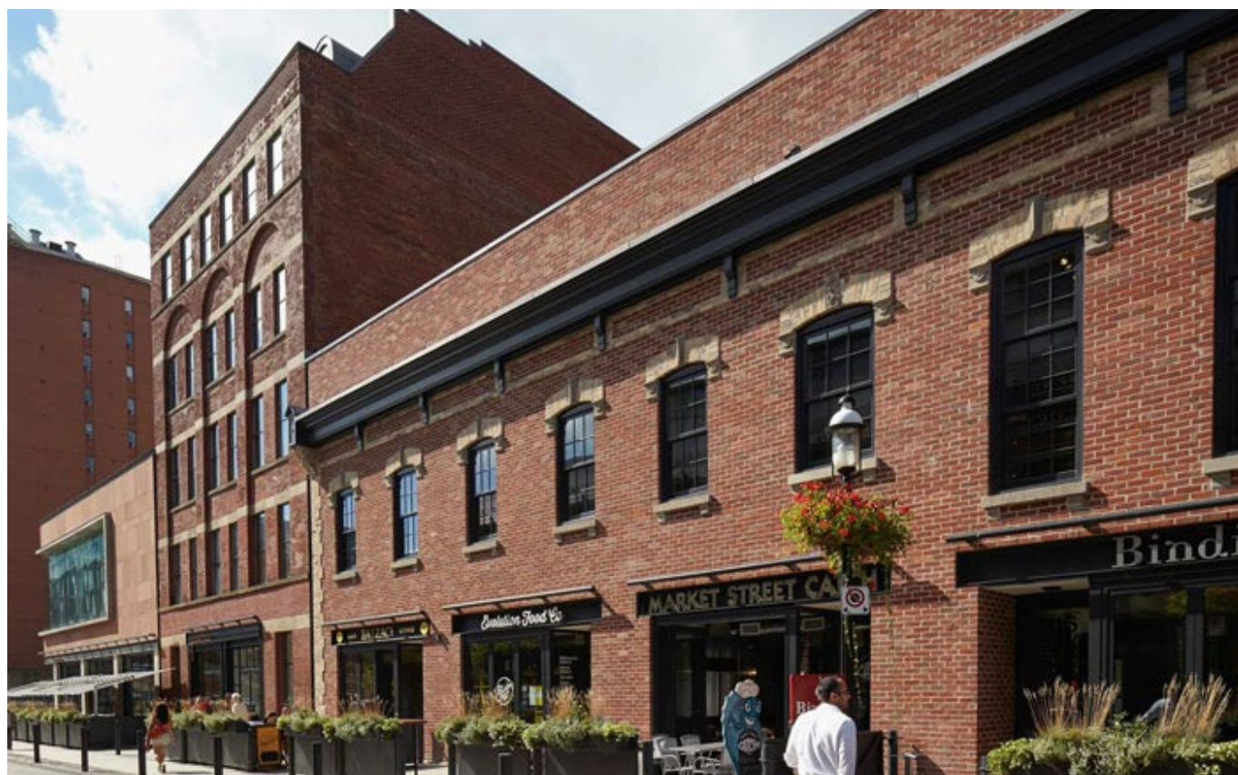
Figure 14: 8-12 Market St., an example of Contributing Properties within the District
