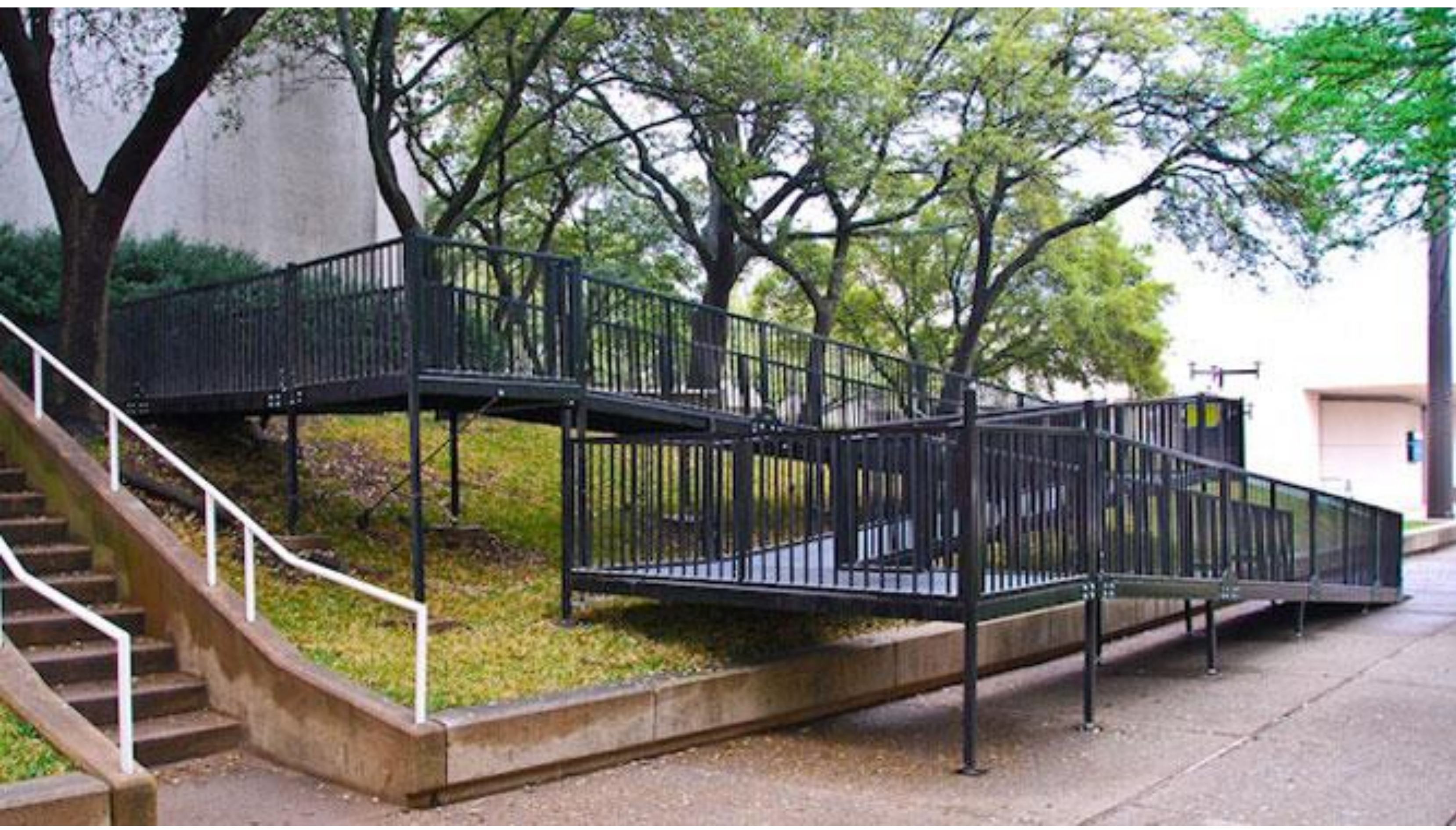
Example of a switchback ramp Source: http://www.portawalk.com/tas_guidelines.html
