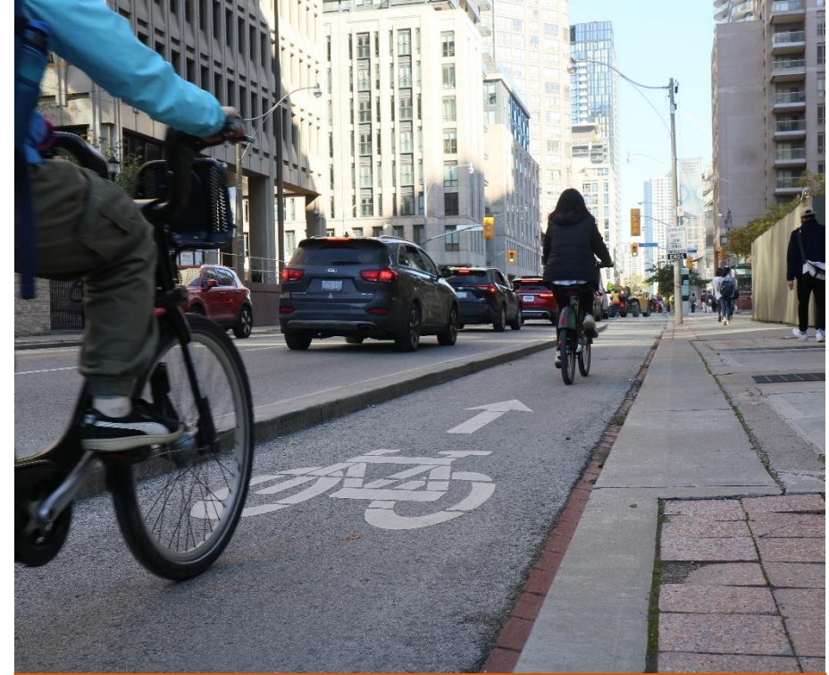
Cast-in-place curb separation on Wellesley Street near Bay Street
