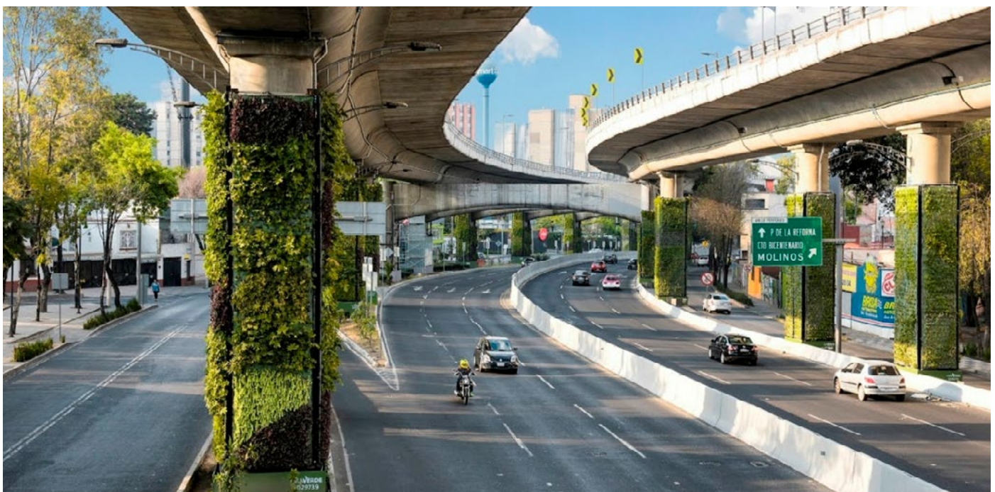
Figure 36: Vertical gardens were constructed on approximately 1,000 piers all along the guideway and other transit infrastructure, Mexico City (Photo Credit: Via Verde)
