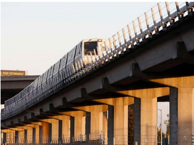
Figure 17: BART Train guards and railing as integrated part of the guideway's design expression, West Oakland (Photo Credit: Michael Short, The Chronicle)
