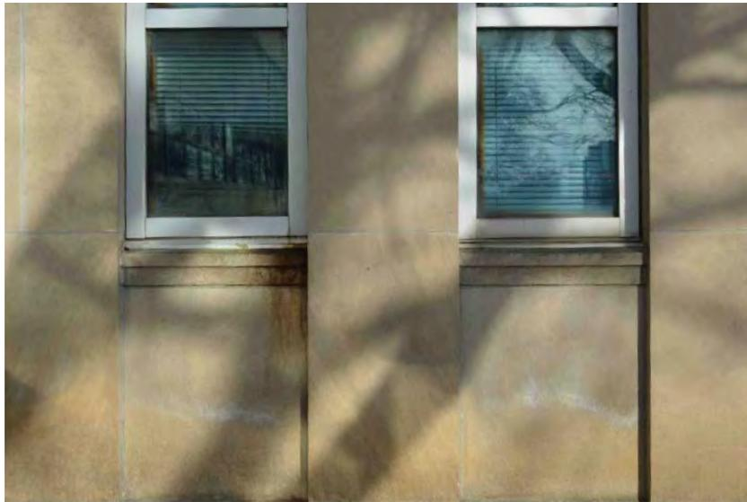
*Salt and rust staining is evident on the wings of the limestone portal entrances*
