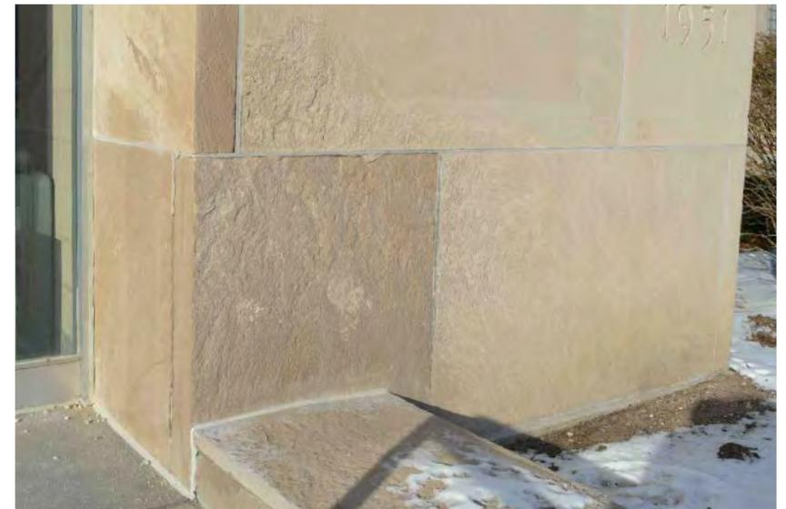
*Erosion evident at grade level of the north portal. Likely caused by ingress of moisture and de-icing salt due to the porous nature of limestone.*
