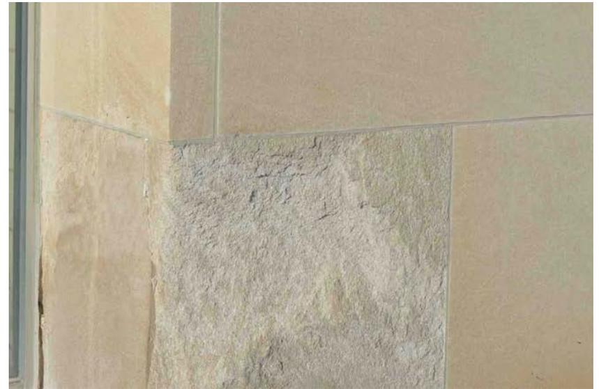
*Deterioration evident at the base of the south portal. Likely cause is de-icing salt and moisture.*
