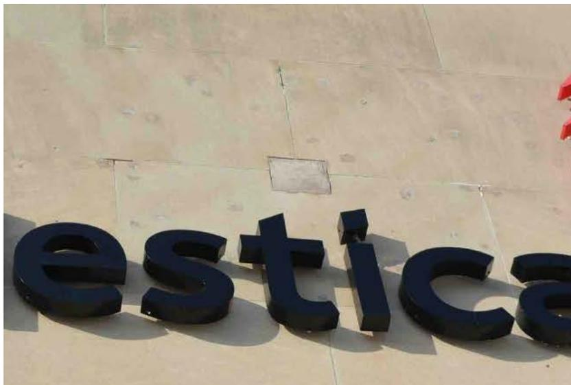
*Previous patch work covering penetrations for the original IBM clock are evident.*
