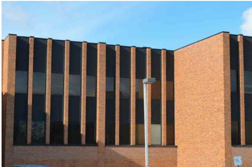
*Replaced brick show white replacement pointing on north elevation below window sill.*
