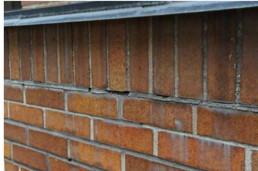
*Detail of brickwork under parapet flashing showing signs of cracked mortar and efflorescence.*
