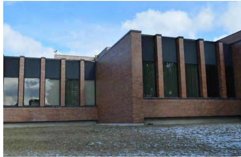
*Efflorescence visible on the south elevation, particularly under window sills.*
