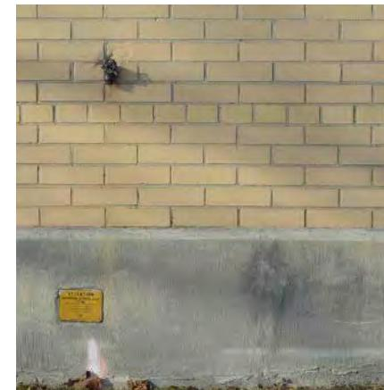
*Staining, spray paint, and penetrations to the masonry units are visible on the east elevation.*
