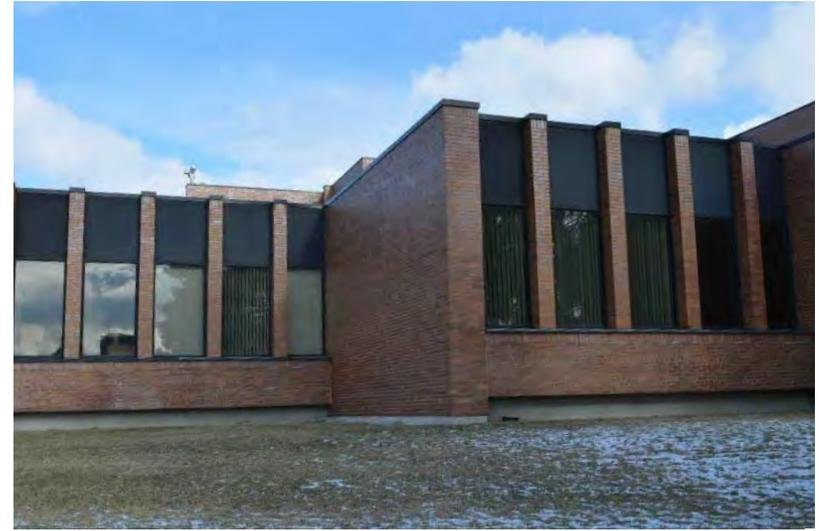
*Efflorescence visible on the south elevation, particularly under window sills.*
