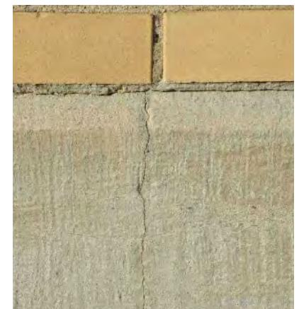
*Crack evident in cementitious parging location the east foundation wall.*
