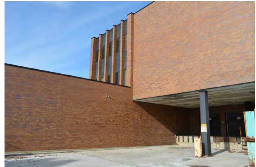
*Control joints seen on the north east elevation, where the two volumes intersect for a loading bay.*
