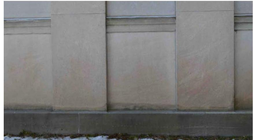
*Organic deposits are evident along the base of the plinth on the elevations of the secondary wings of the entrance portals.*
