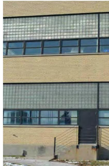
*View of the east elevation. The concrete stairs are heavily stained by rust.*
