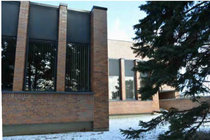
*Replaced and discoloured masonry visible below the window on the south Elevation.*
