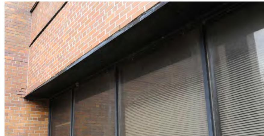
*Detail of a lintel over a window opening at the south elevation. Notice the recessed mortar joints at the intersection of both walls, on the left.*
