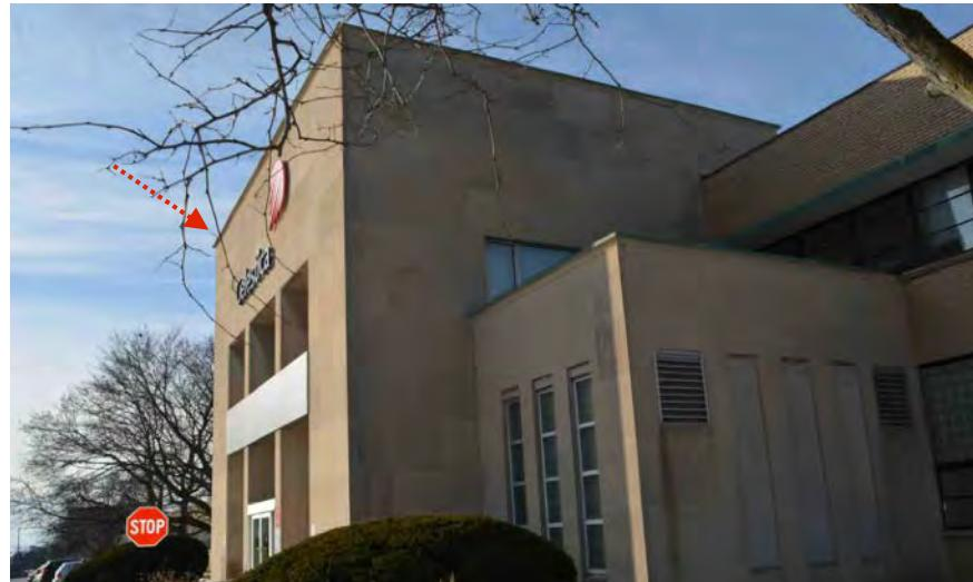
*View (looking south) of the northern entrance portal fronting Don Mills Road. A recessed joint and displaced stone was noted near the parapet (arrow). Note the staining evident on the limestone wing, as a result of the metallic venting and exhaust.*
