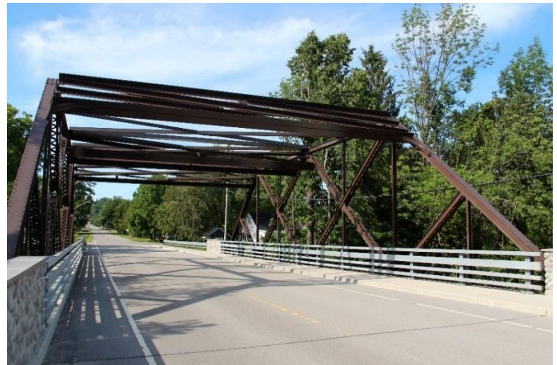
New Creemore Bridge, Clearview Township, ON (Source: https://www.flickr.com/photos/cmhpictures/36341729453 )
