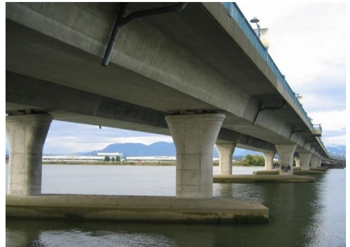
No. 2 Road Bridge, Richmond, B.C. (Source: Homelist Vancouver, n.d.)
