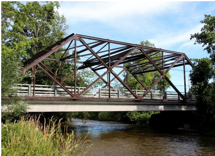
New Creemore Bridge, Clearview Township, ON (Source: https://www.flickr.com/photos/cmhpictures/37155082985 )
