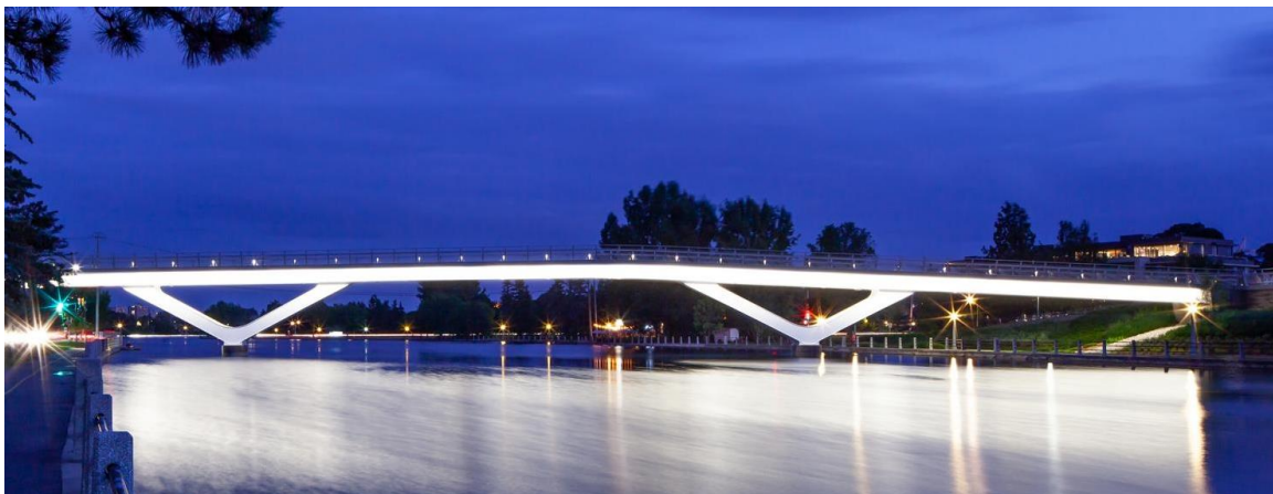
Flora Footbridge, Ottawa (Source: https://dtah.com/work/flora-footbridge )
