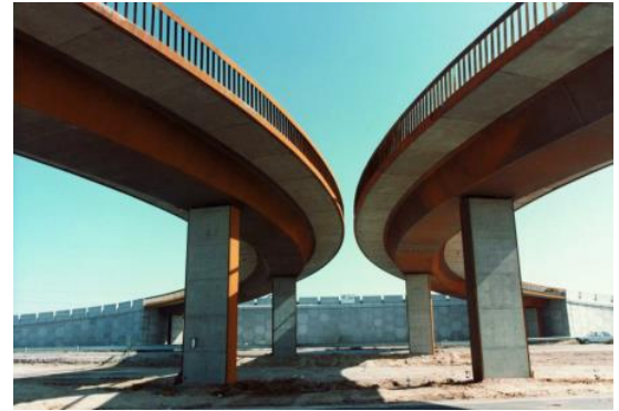
N-II Motorway, Madrid, Spain (Source: https://www.mc2.es/en/proyect/bridge-access-pryca-a-2 )
