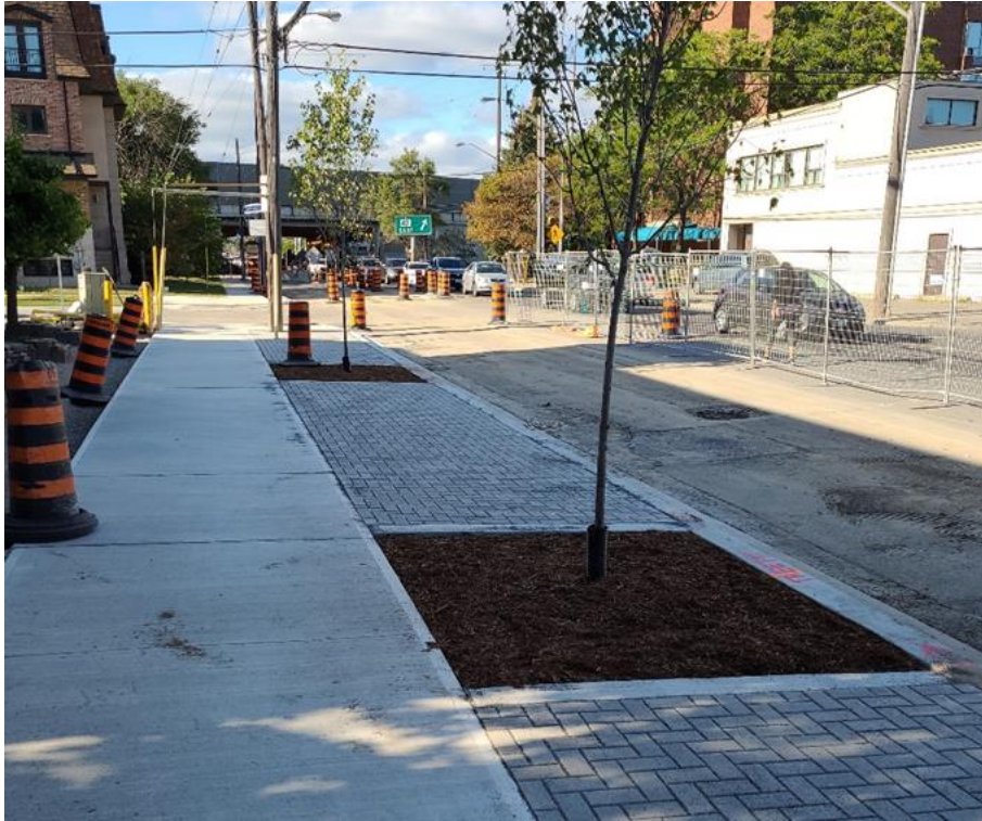
Planned tree openings and permeable pavers
