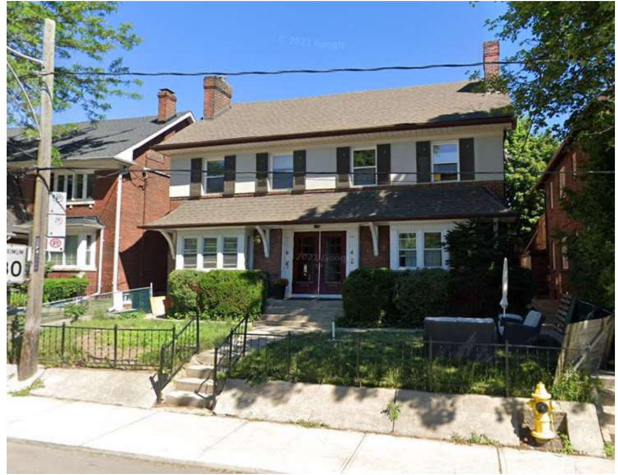
Semi-detached houses on College View near Oriole
