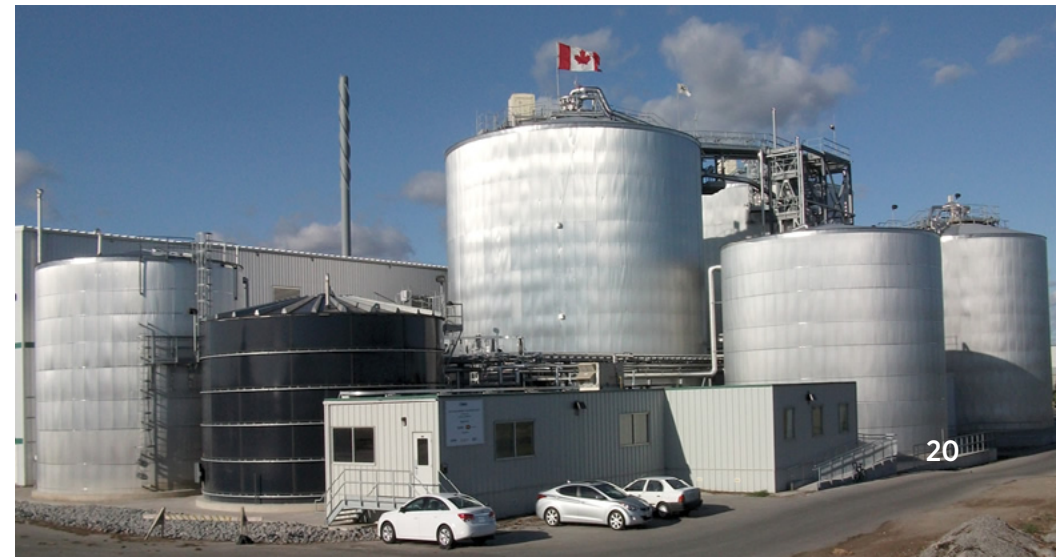
Dufferin Organics Processing facility
