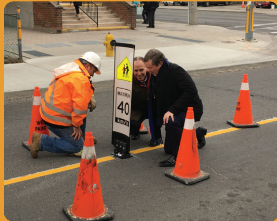
Councillor Josh Colle and Mayor Tory on hand for the installation of first sign as part of a pilot on March 27, 2018.
