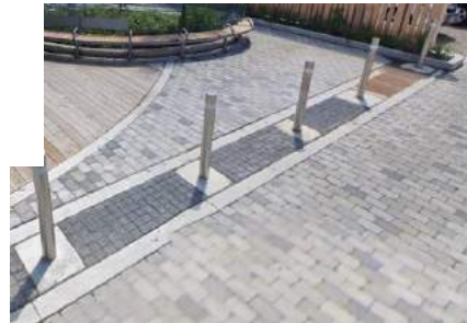
Image of Glasgow Street, east of Spadina Ave and Oxford St
