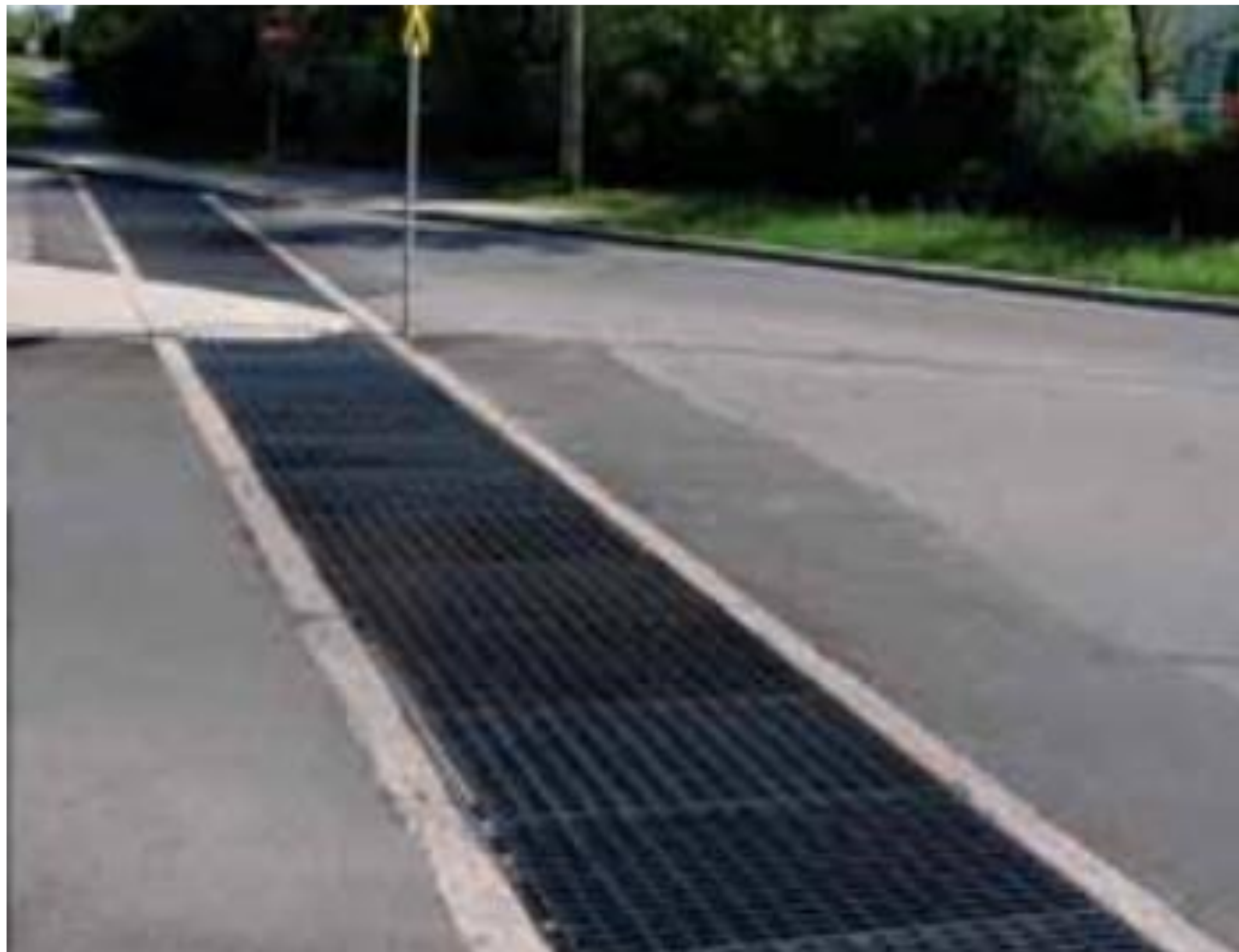
Example of a high-capacity inlet*
