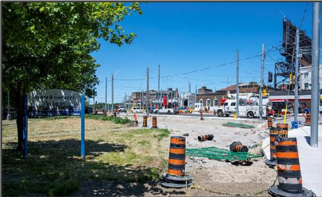
Expansion of Beaty Boulevard Park Underway
