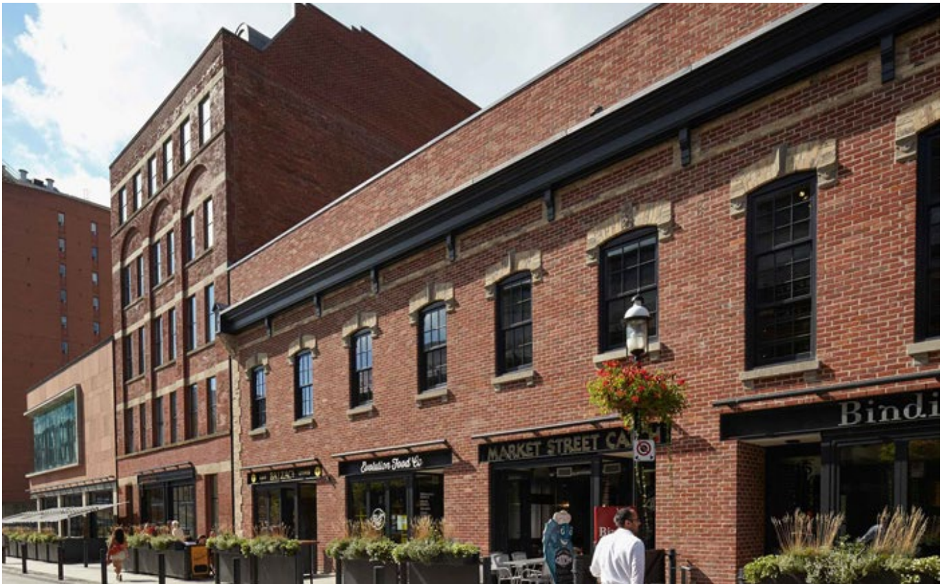
Figure 14: 8-12 Market St., an example of Contributing Properties within the District
