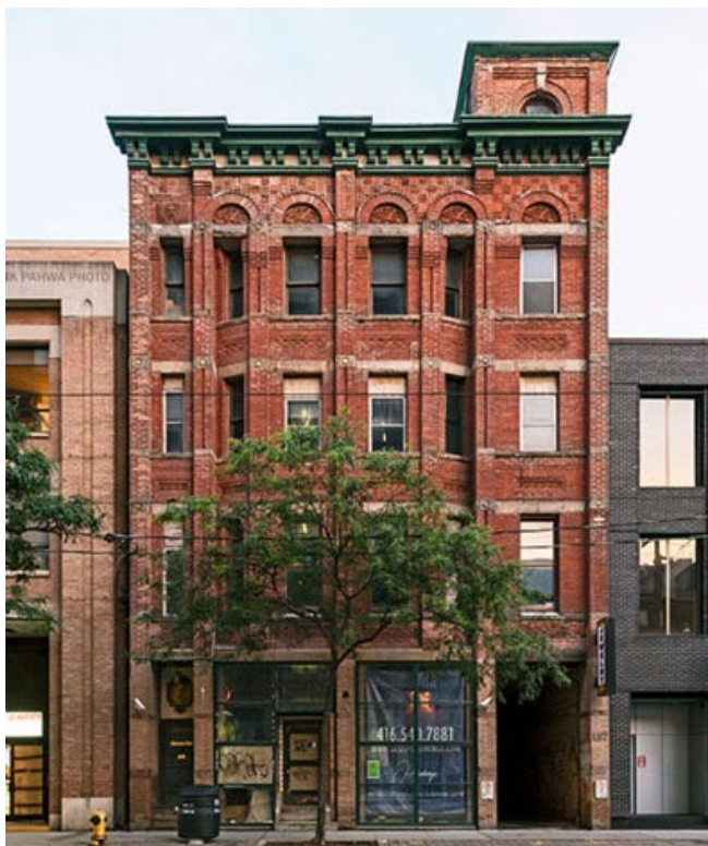
Figure 5: 197 King St. East, also known as the Nealon House, dates to 1888 and displays many decorative elements typical of the late Victorian era, photographed by Vik Pahwa
