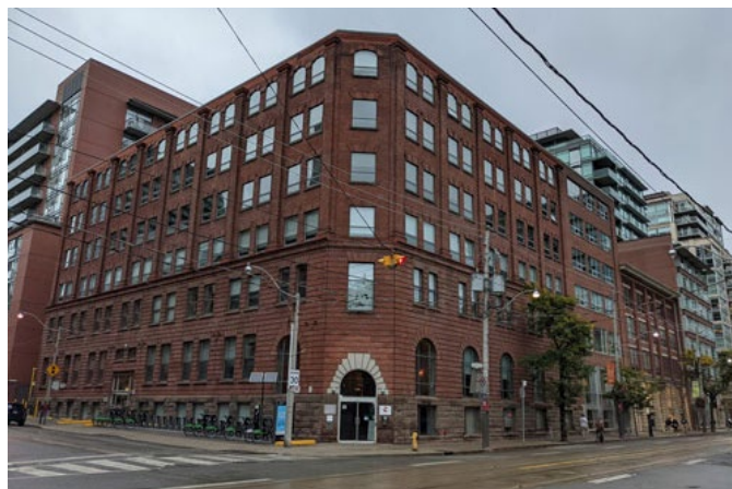
Figure 12: 204 King St. East, an example of Industrial Building Typology
