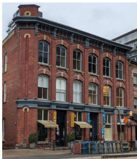
Figure 7: 67-69 Front St. East, an example of Commercial Warehouse typology
