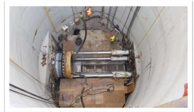
Image: inside of the vertical shaft
