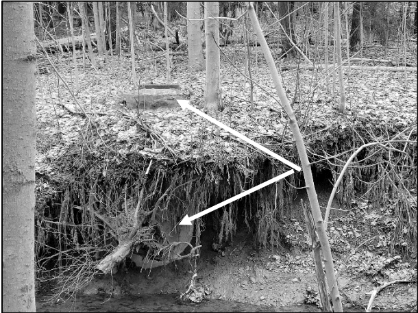
Exposed manhole in the bank
