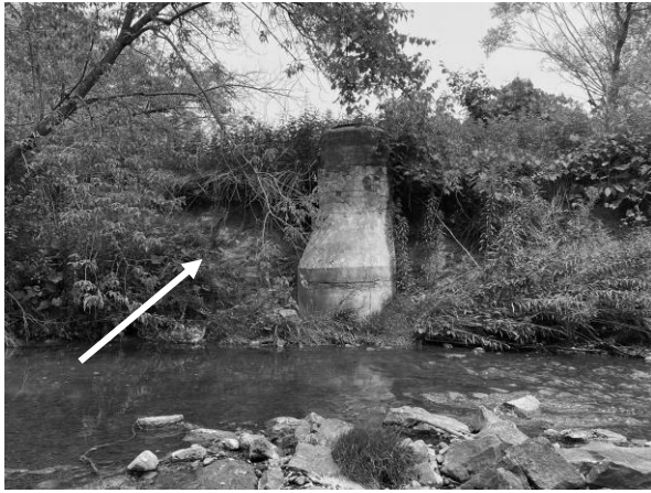
Exposed Sewer Manhole
