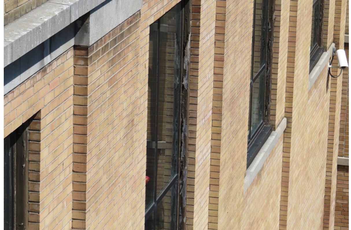
Image description: Deterioration of wood window frames
