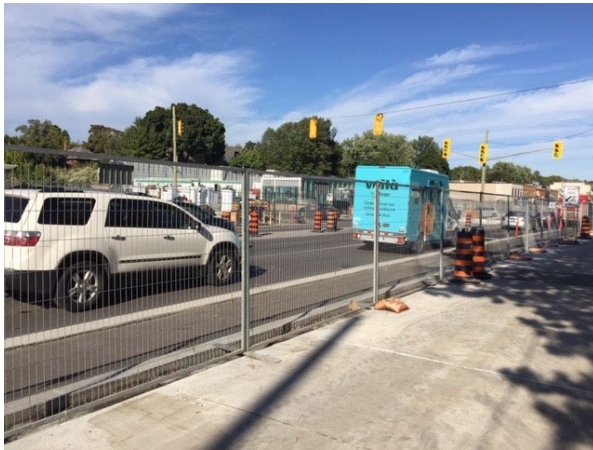
Sidewalk Fix, Marlee Ave to Bathurst St Site Walk, Sept 21, 2022.
