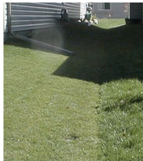
Improving lot grading
