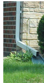
Disconnecting downspouts
