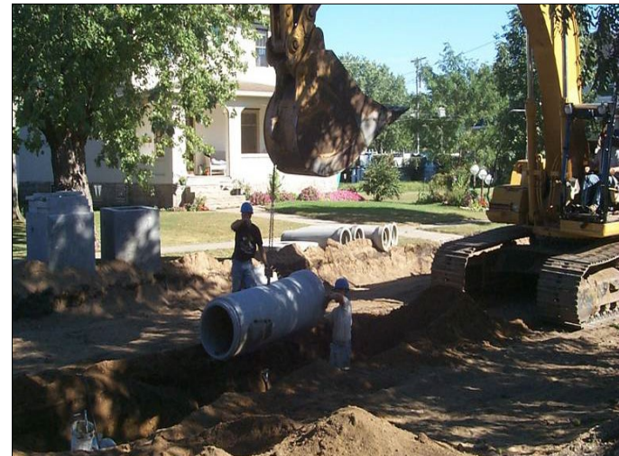
Image of storm sewer replacement in road during construction
