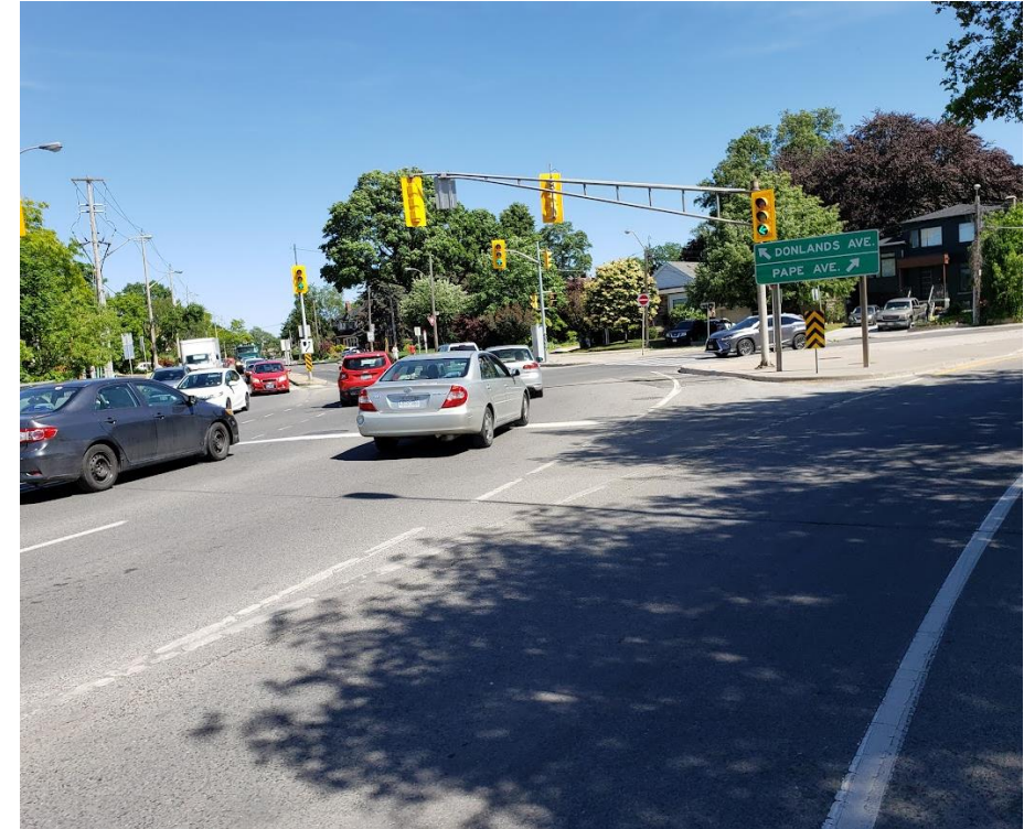
Missing crosswalk of Pape Avenue and Millwood Road
