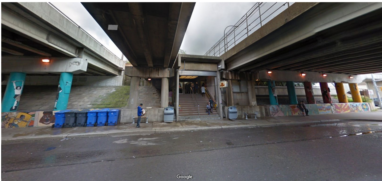
Figure 4-60. Yorkdale Station Subway North Entrance from Yorkdale Road
