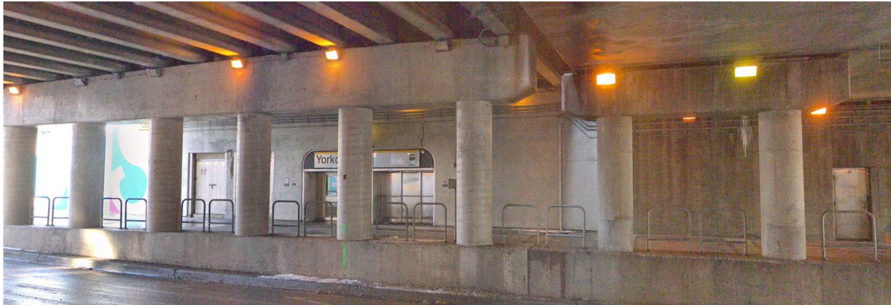
Figure 4-61. Yorkdale Subway Station South Entrance from Ranee Avenue
