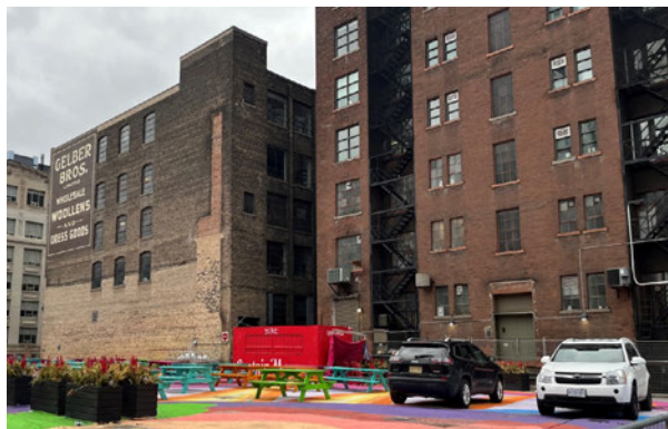
East side of the site showing the Gelber building and the Caplan building
