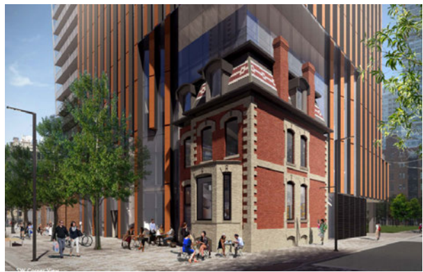
View from southwest of proposed 241 Richmond Street West development showing integration of heritage building at 133 John Street (architects-Alliance)
