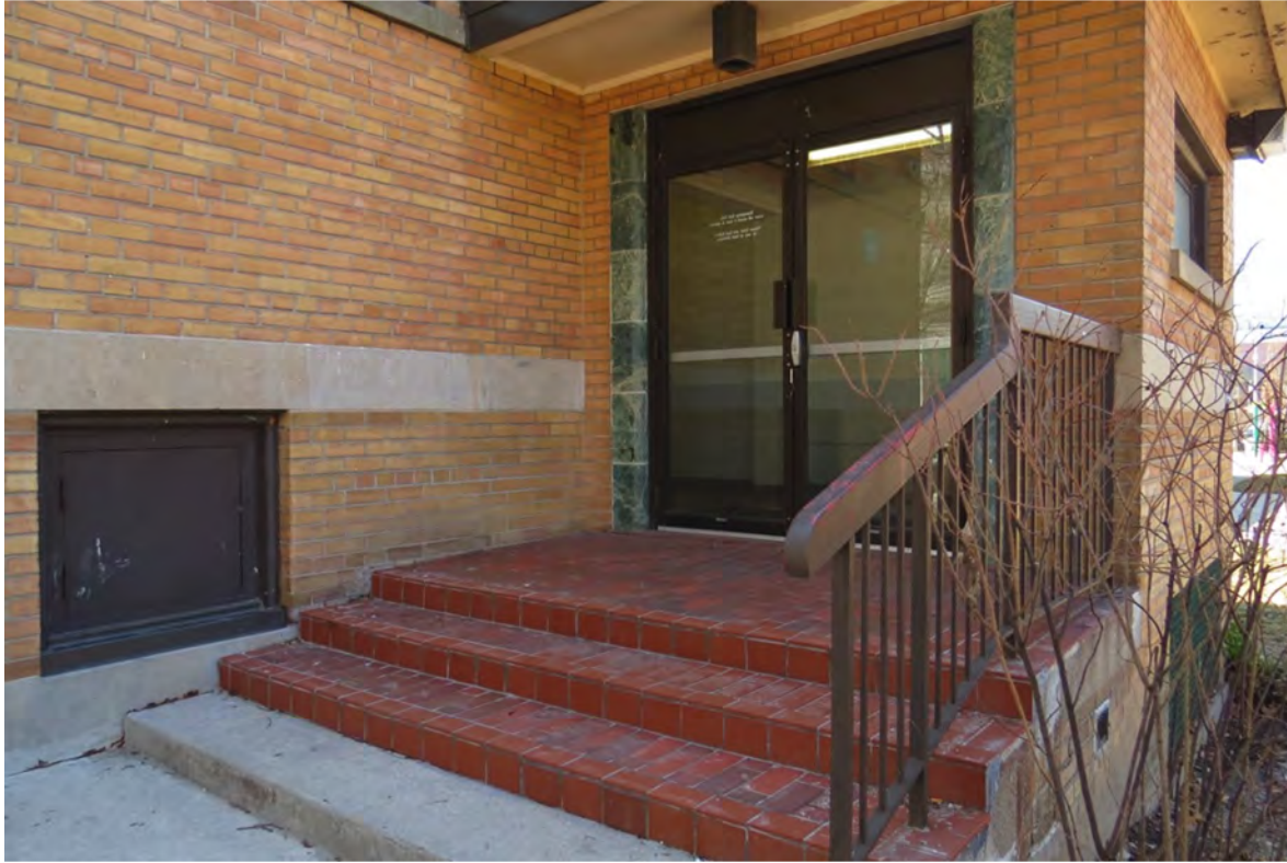
Image description: Non-AODA compliant entryway/exit to the John Innes Community Recreation Centre
