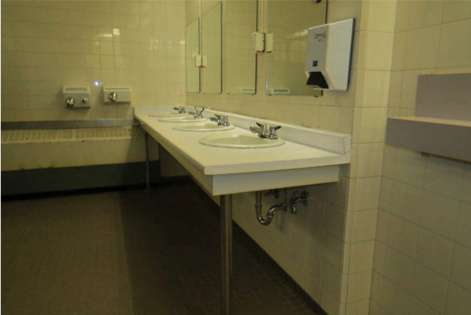
Image description: Existing hand washing areas in the washroom
