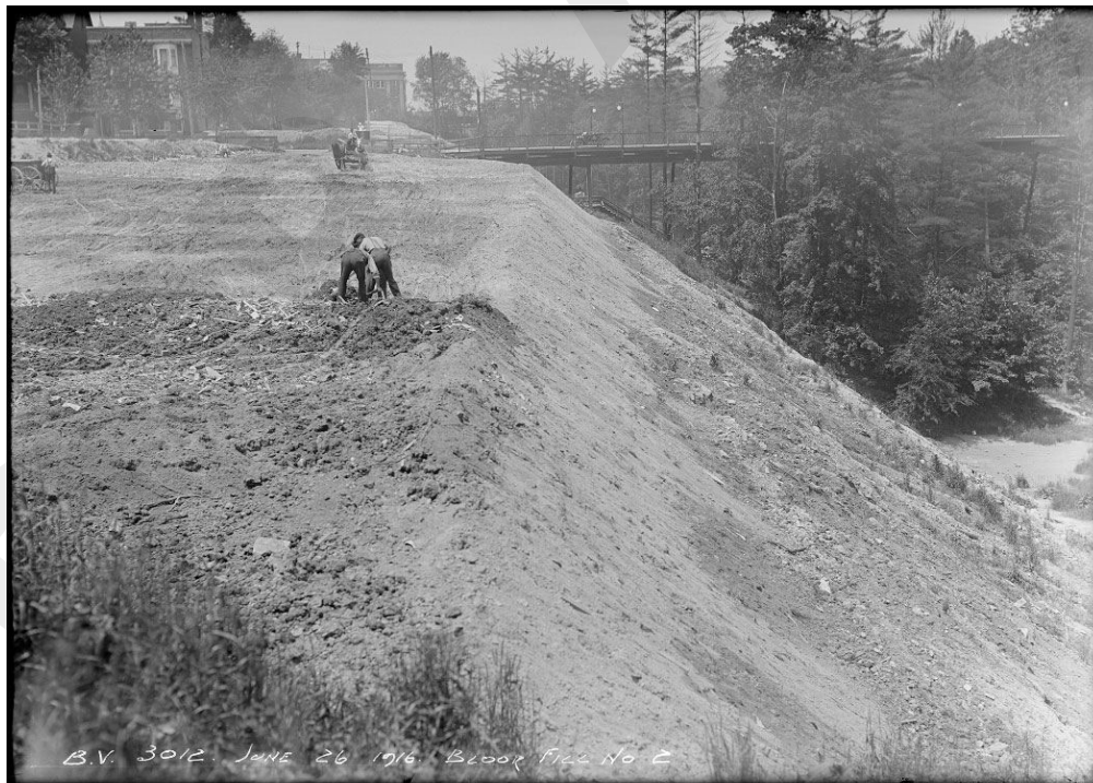
Figure 22: 1915 archival photograph looking northeast to Bloor and Sherbourne streets, with the Toronto Dominion Bank building in the background. In the foreground an embankment is being build-out over the Rosedale Ravine to support the extension of Bloor Street East ( City of Toronto Archives ).
