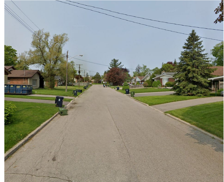
Existing Conditions on Penetang Crescent
