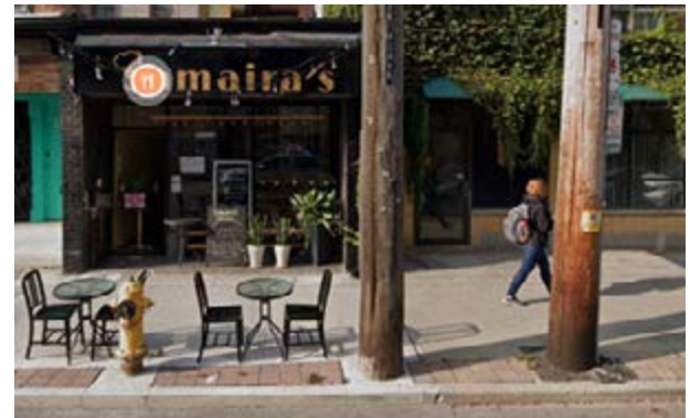
Distribution/Street Lighting Pole
