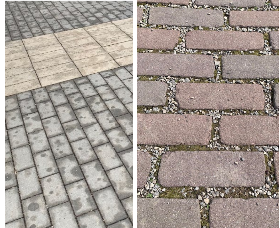
Permeable unit pavers at Dundas Street East and River Street (left), and Bremner Boulevard at Steam Whistle Brewery (right)
