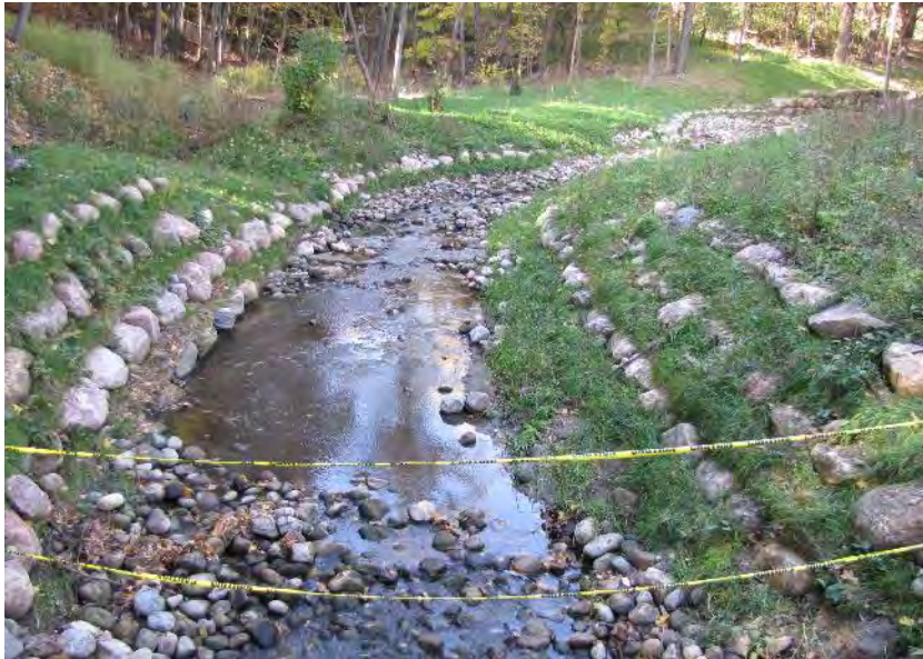
Mud Creek: Stream bank constructed with a vegetated stone buttress
