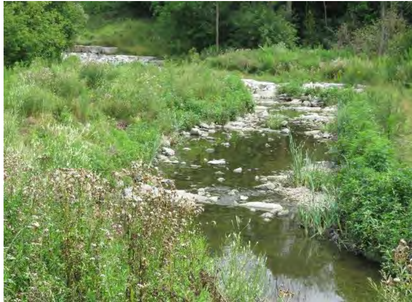
Berry Creek: Stream realigned and bends to move away from previously exposed sanitary sewer crossing
