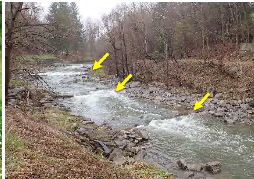
West Highland Creek: Rock weirs allow for grade control that reduces flow speed, provides pool and riffles, and stabilizes stream bed material.
