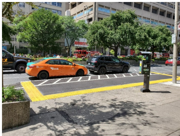
Figure 10: On University Avenue near a hospital entrance, Transportation Services installed an accessible platform to create barrier free access. This by-law would require people cycling to yield to people with disabilities being picked up/dropped off.
