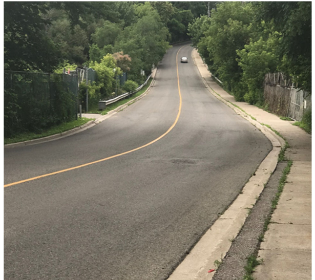
Figure 5: Scarborough Golf Club Road, south of Confederation Drive, has one motor vehicle lane per direction and minimum-width sidewalks on the east side.
