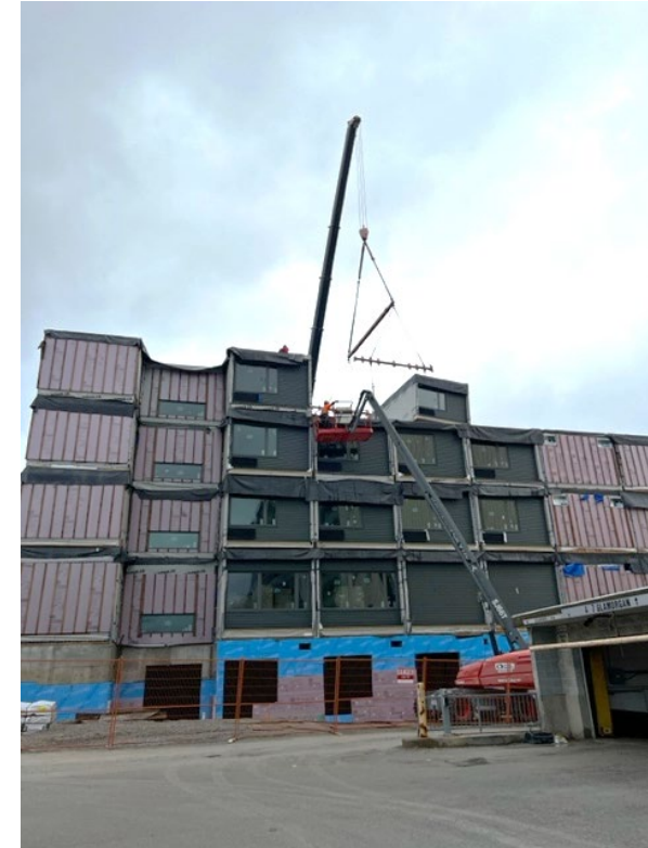
Module craning at 39 Dundalk Drive
