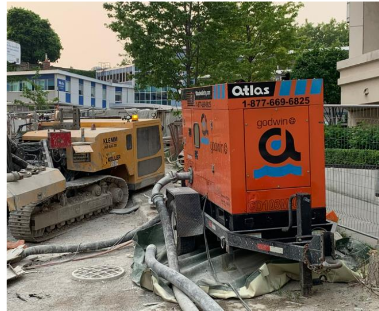
Adjacent to 2 Old Mill Drive
