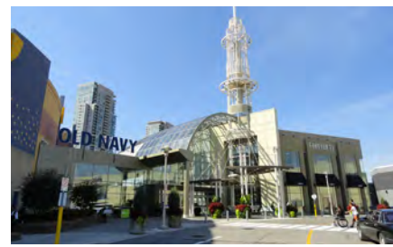
Scarborough Town Centre Mall
