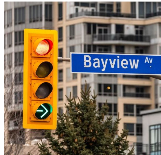
New Traffic Signal
