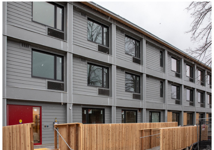
Modular building at 321 Dovercourt Rd.
