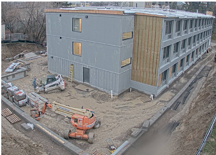
Construction of modular building
