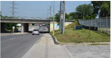
Pedestrian sidewalks located directly next to high speed/high volume traffic lanes due to lack of furniture/buffer zone
