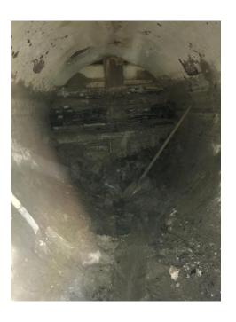
• The Contractor is now preparing the bottom of the shaft, including breaking out and replacing the mud slab, which is essentially a layer of concrete that is poured over the muddy soil at the shaft's base to create a foundation for constructing a reinforced floor slab. This floor slab will be equipped with an anchor system that is necessary for the extraction of the Micro Tunnel Boring Machine (MTBM).
