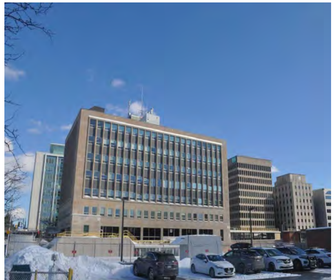
Image 3. View of McBrien Building from Chaplin Crescent towards Yonge Street
