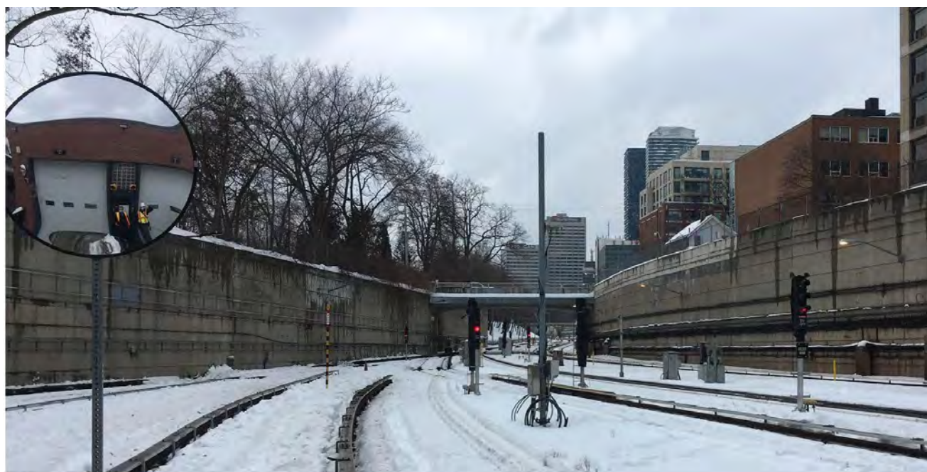
Image 40. TTC Trench facing North
