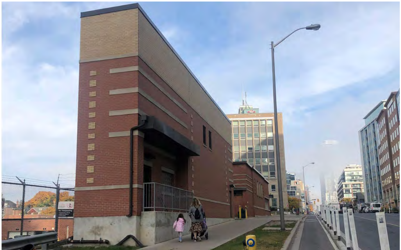
Image 55. Signal Control Building
