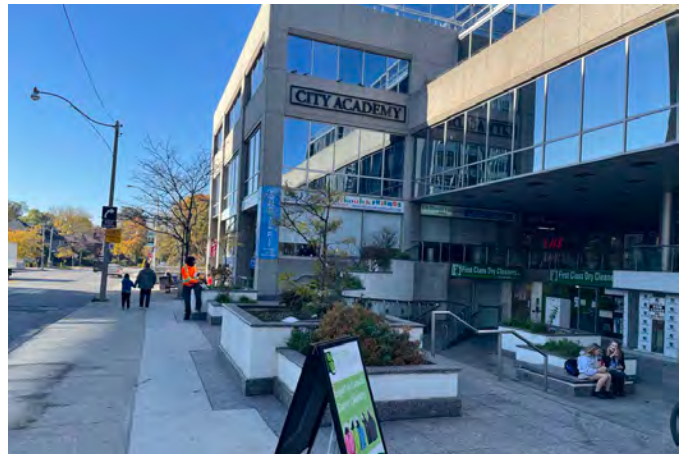
Image 83. View of the semi public plaza at the intersection of Chaplin Crescent and Yonge Street
