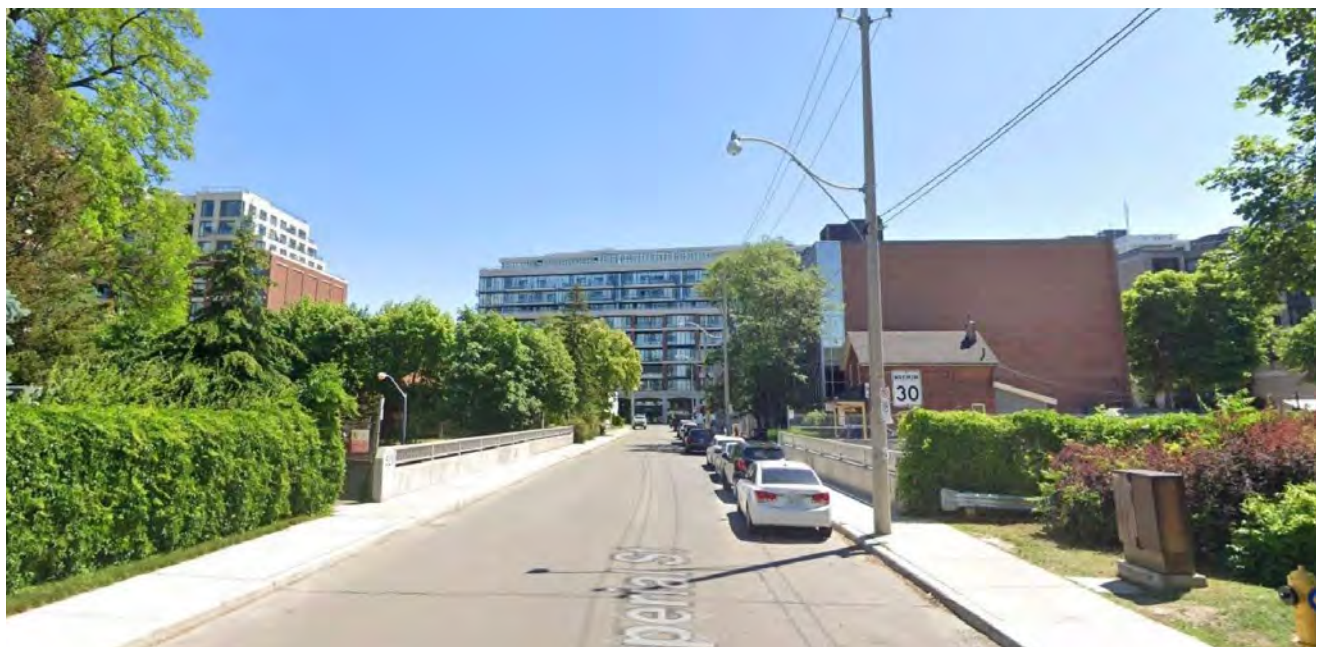
Image 39. Imperial Street Bridge facing East
