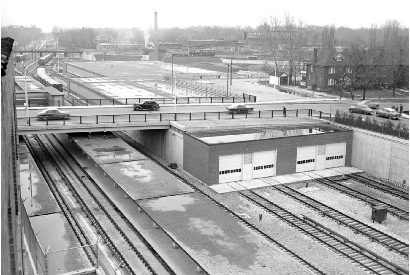
Image 63. View of the Davisville Yard and Shop Building (at the right), looking south. November 24, 1953
