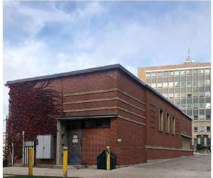
Image 5. Traction Substation Building
