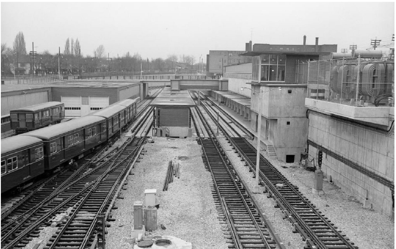
Image 64. View of the Davisville Station looking North, 1953
