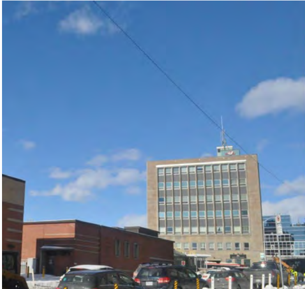
Image 4. Traction Substation Building
