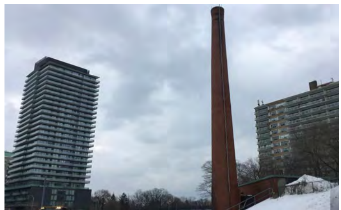
Image 10. Davisville Boiler House Chimney
