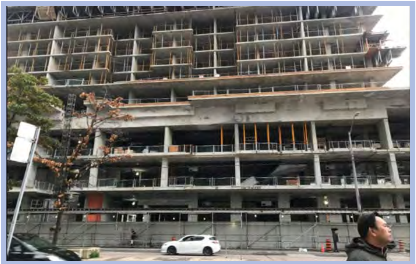
Figure 15.1 – Active construction project on Yonge Street
