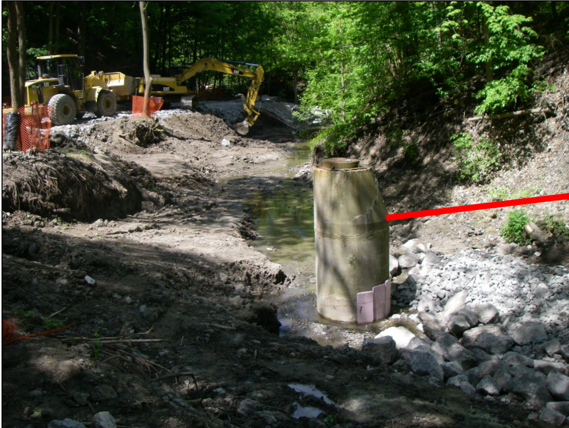
Massey Creek - Sanitary sewer maintenance hole within the creek channel (during-construction)
