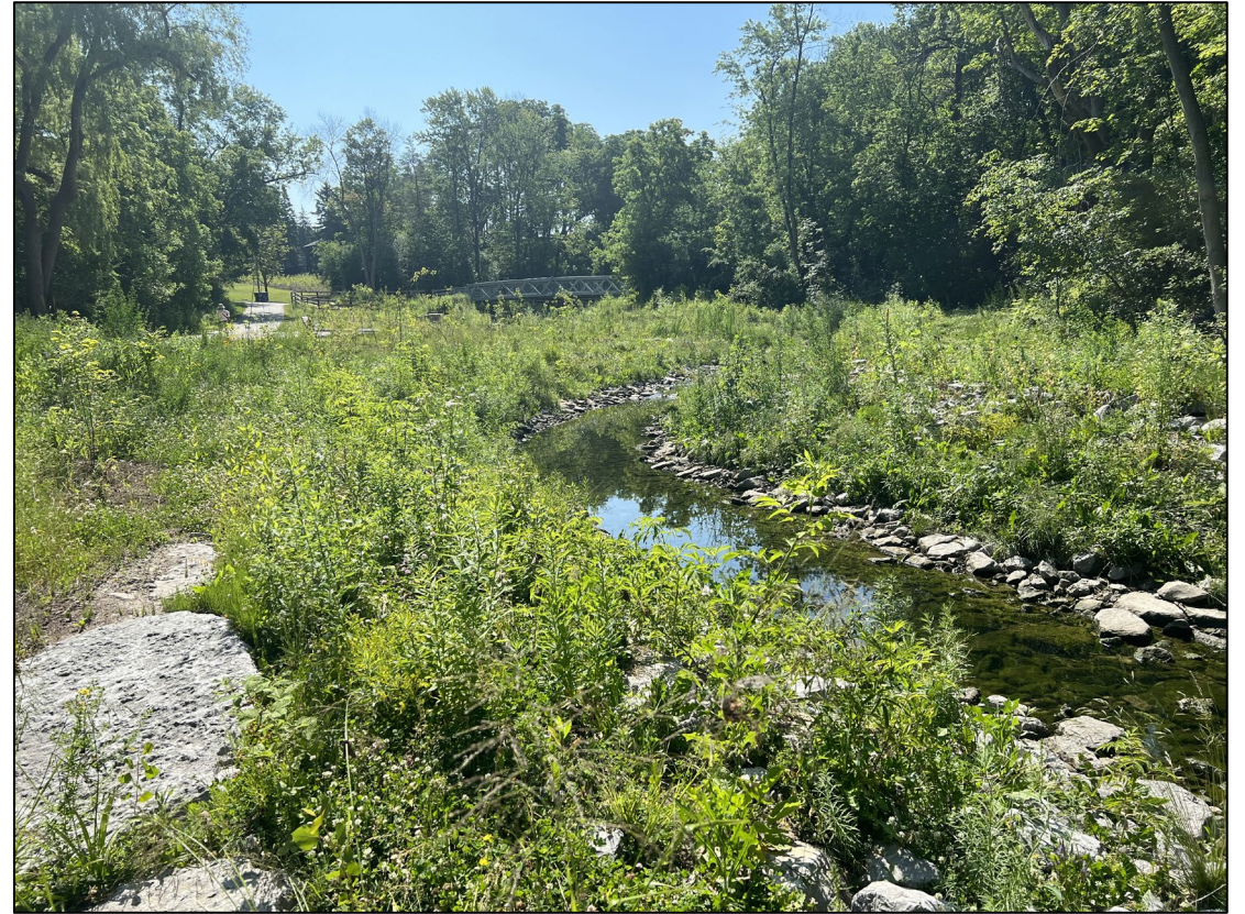
Duncan Creek Phase 2 – Rehabilitated creek corridor (post-construction)
