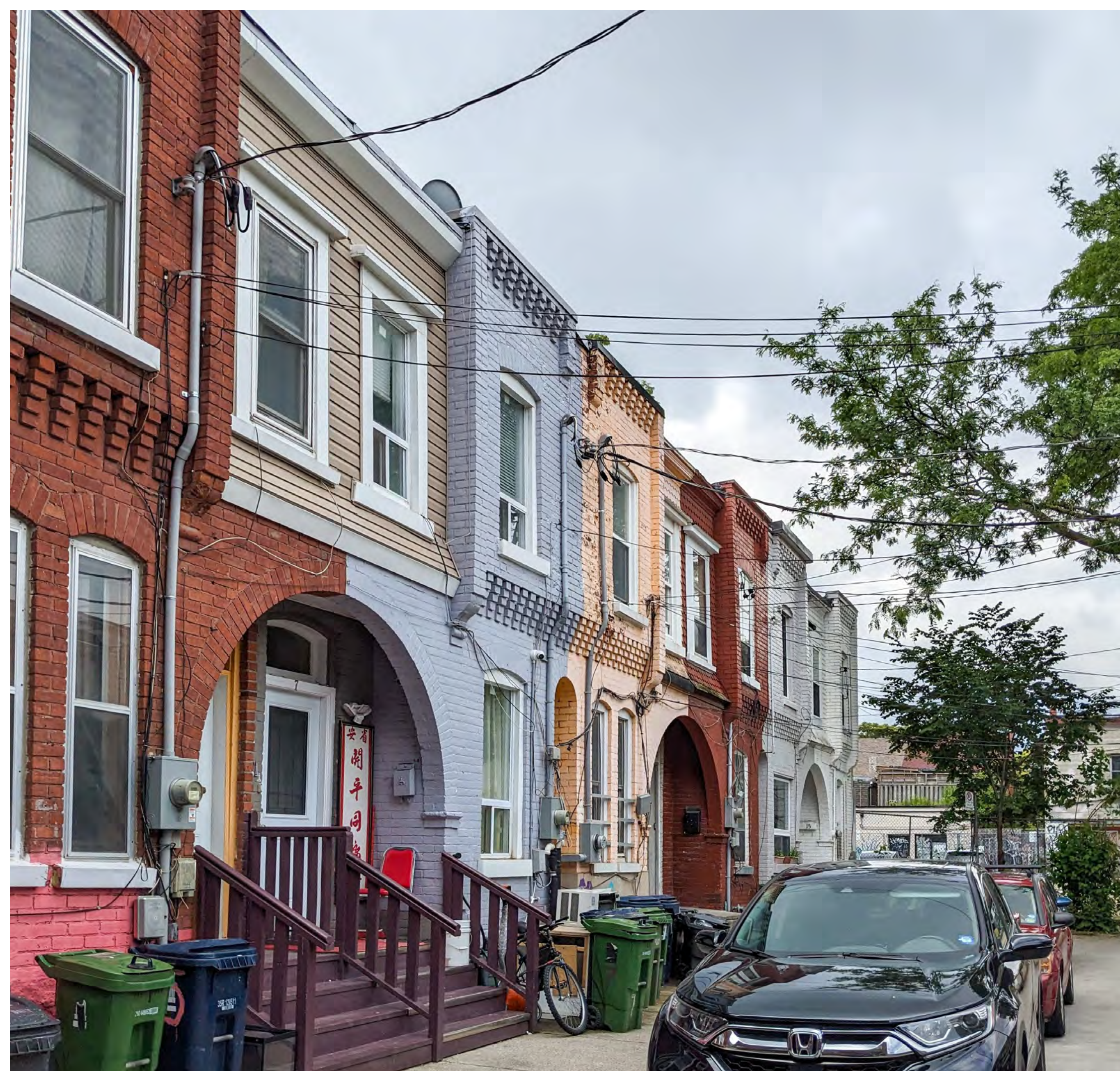
Façade materials | Horizontal siding has replaced wood shingles above the entrances to 5 & 7 Glen Baillie Place
