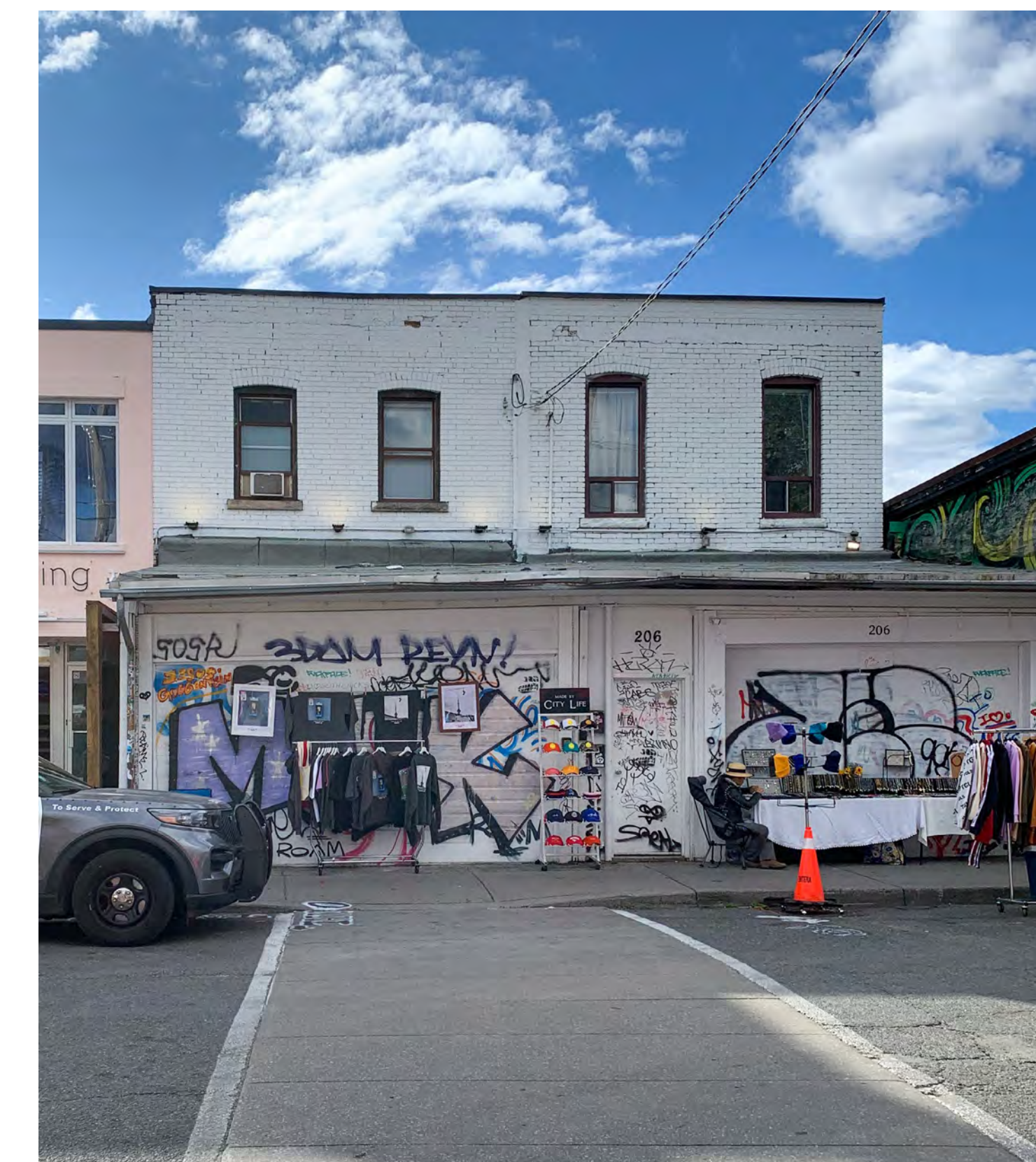
Commercial | The properties at 204-206 Augusta Avenue are examples of the commercial typology
