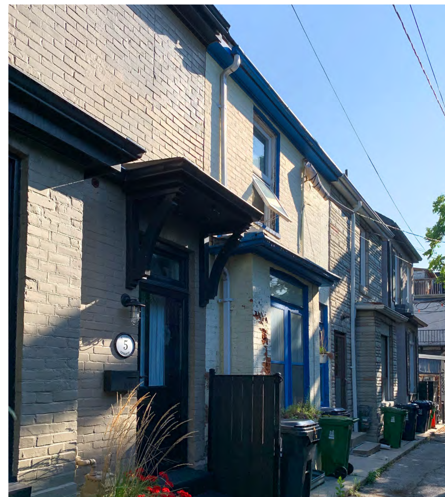
House-form – Row | The laneway housing at 5-8 Fitzroy Terrace is an example of the House-form building typology configured as a row
