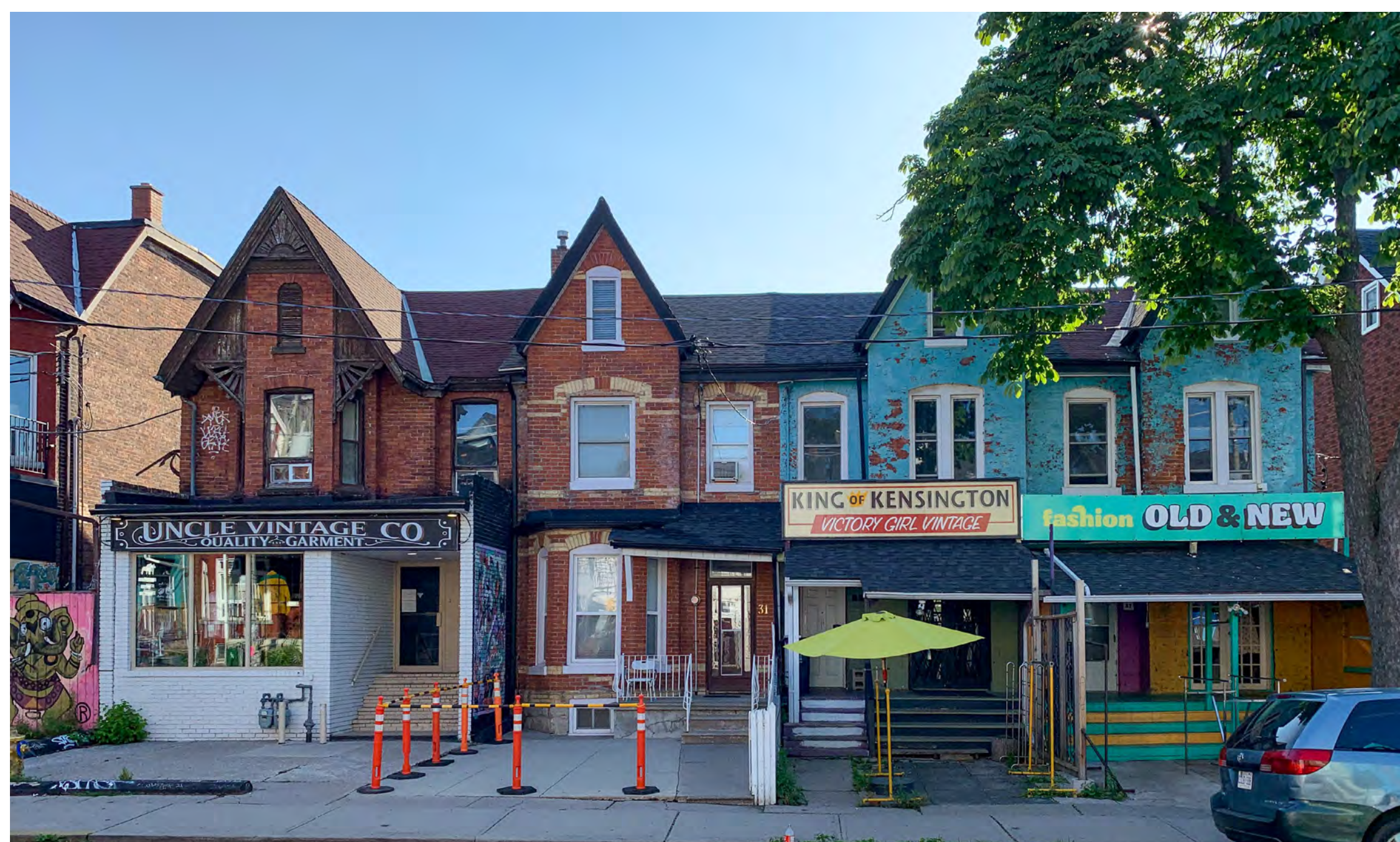
Front Additions | Many properties within the Commercial Market have existing one-storey additions in the front.
