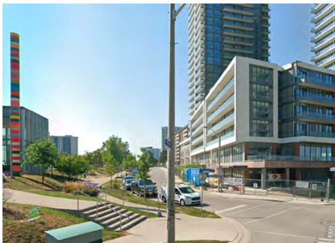
Towers and base buildings should be shaped, located, and oriented to preserve comfortable conditions for pedestrians, with consideration for microclimate (wind and sun) – Forest Manor Road, Toronto
