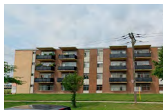
Existing low rise apartments that are typically 'slab' type buildings
