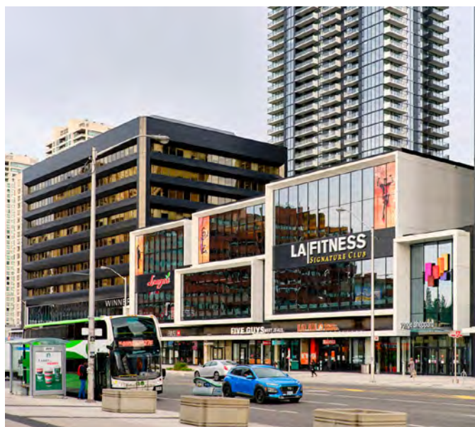
Yonge-Sheppard Centre features taller storey heights to accommodate non-residential uses such as supermarkets, restaurants, gyms, and retail (Archilovers)
