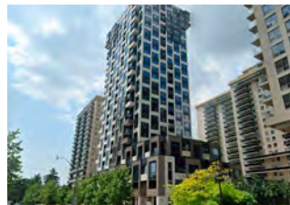
Example of a tall building (High Park Avenue)
