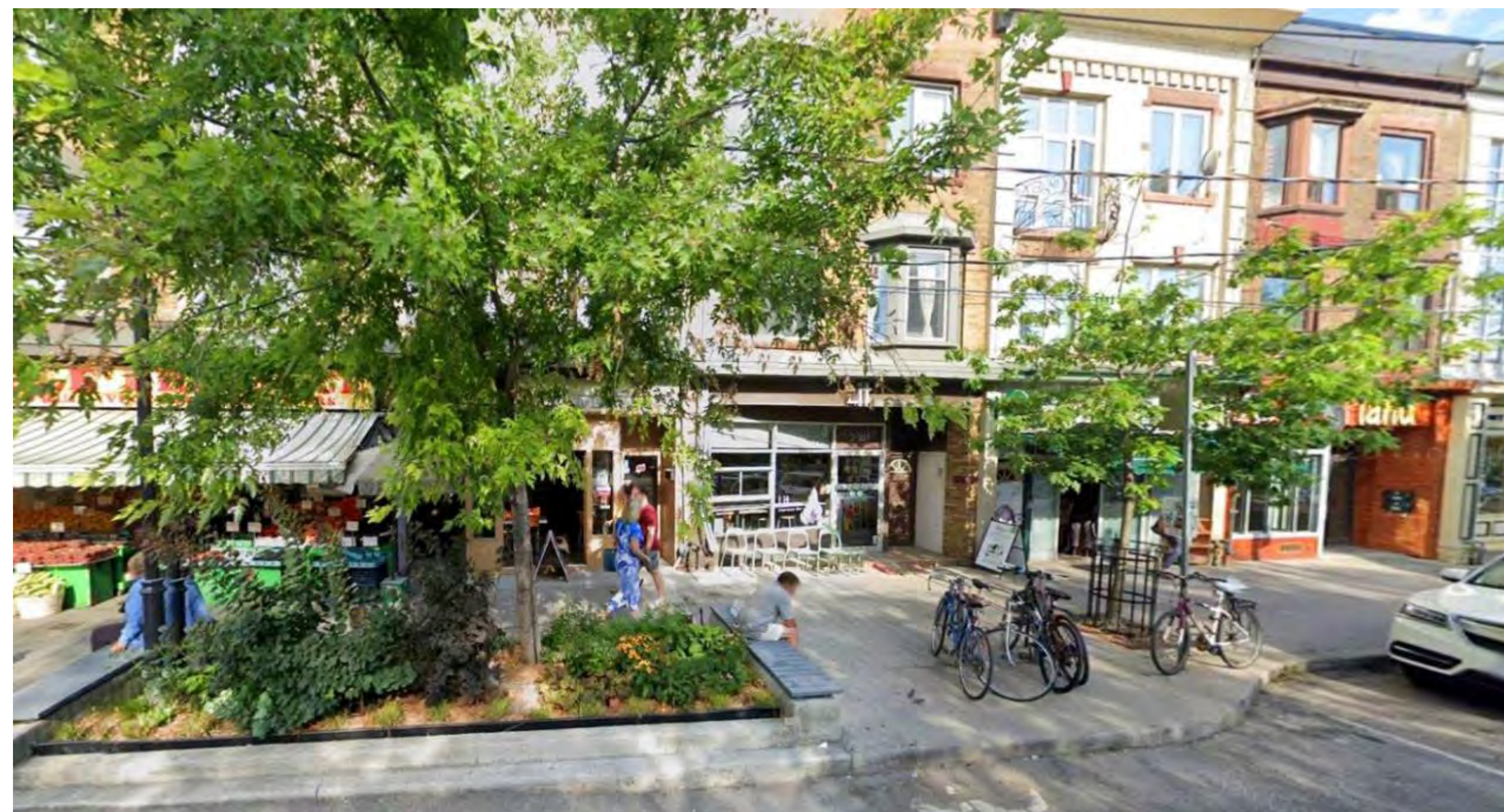
Photo of a bump-out on Roncesvalles Ave to provide room for planting and seating where a few on-street parking spaces had been previously.
